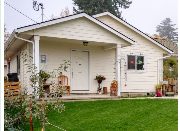
2 nd Street Home Build, 2018
